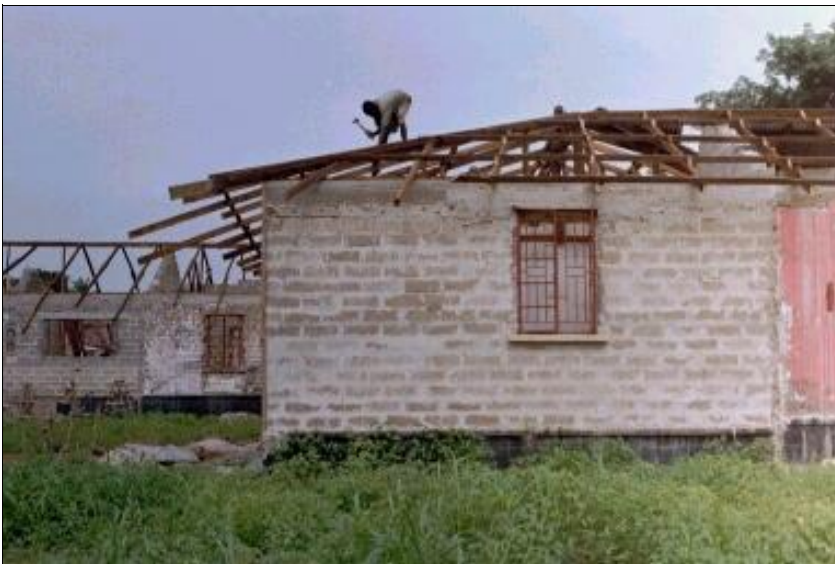
Kambia hospital site
